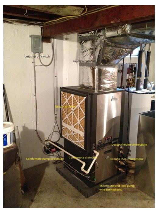
After this it was just a matter of making electrical connections filling the loops purging the air from the system and performing system startup procedures. All went without a hitch system up and operating.
