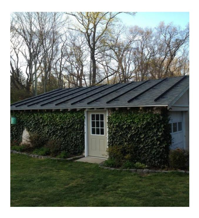
The next morning the panels went up they just plug together in series. The array is split into two separate arrays Right and Left 10 panels each, the inverter has two inputs and controls the outputs separately with individual MPPT.
