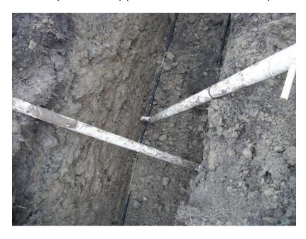
The tools allow the heat pump loop pipes to be positioned without going into the trench and avoid the possibility of being trapped, injured, or killed by a trench cave in.
