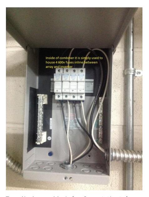
The combiner box opened showing fuses. Fuses protect inverter from over current. There are 4 20 amp 600v fast acting fuses one for each PV array wire to inverter. The PV wires also must be encased in metal conduit from the entrance into any structure to the inverter. Outside can be PVC.
